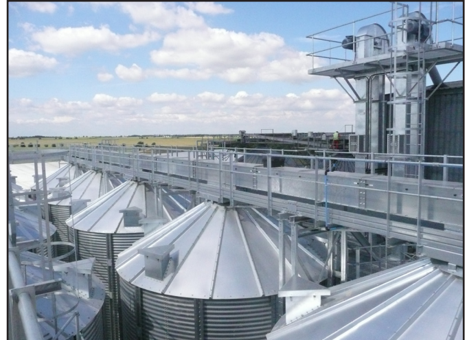
Aerial view of the storage bins and intake system.
