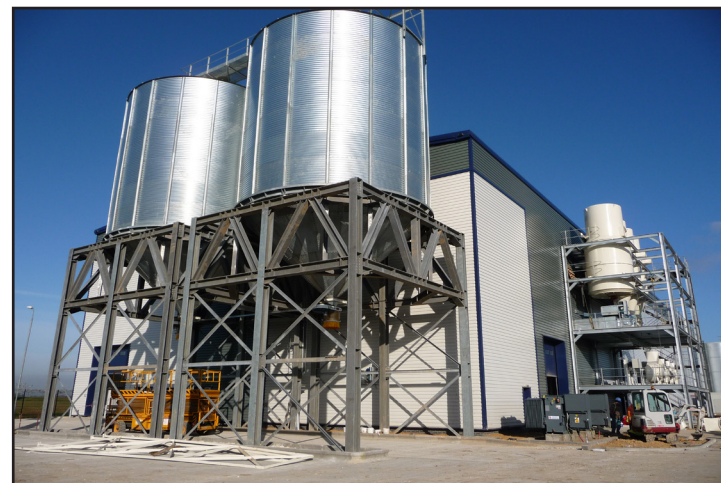
Biomass Bulk Outloading System
